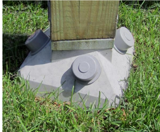
Figure 7. Completed Installation with Pin Caps
