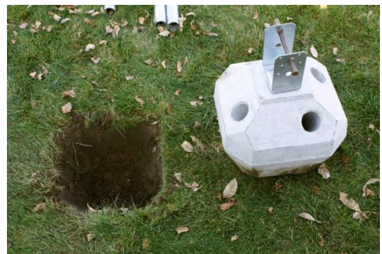
Figure 3. Tapered Hole for Concrete Head
