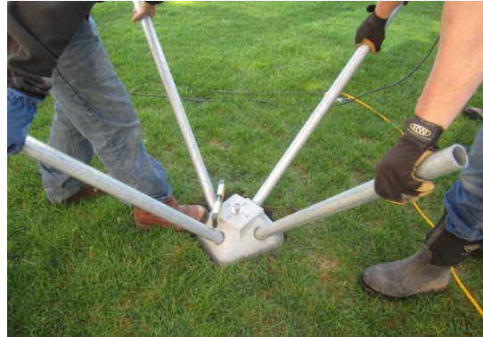
Figure 4. Setting Pins and Leveling Pier
